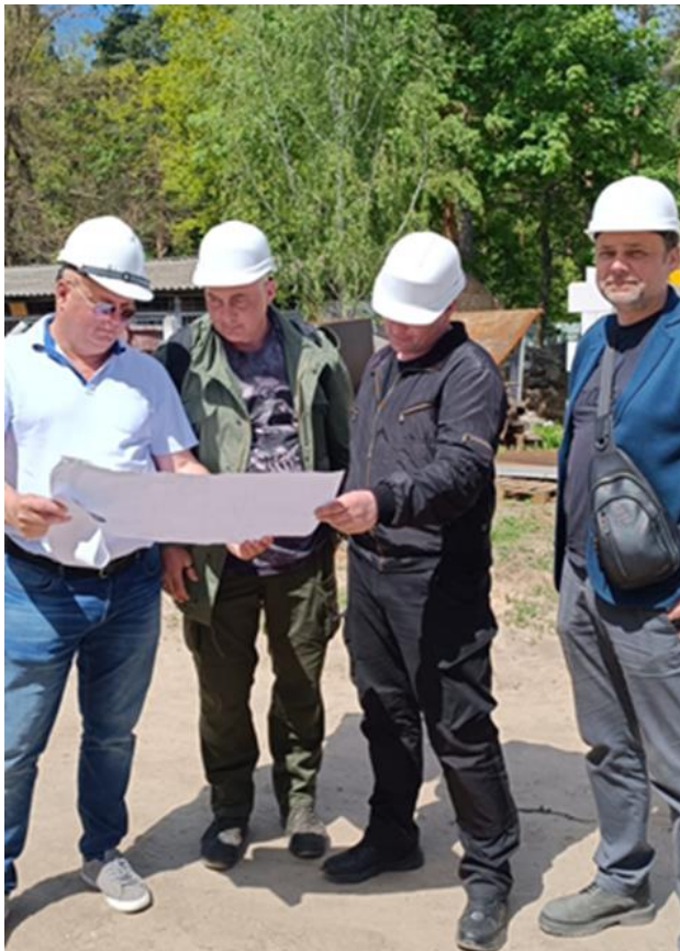
Assessment of a damaged facility in Kyiv lead by Oleh Vasenov
